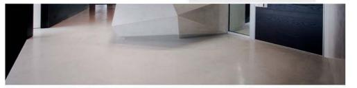
MICROCEMENT: ideal for those seeking a continuous, textured finish, with a thickness of just 3 millimetres. Microcement allows for the renovation of various existing surfaces — such as concrete, ceramic or wood — with no need to removal.
